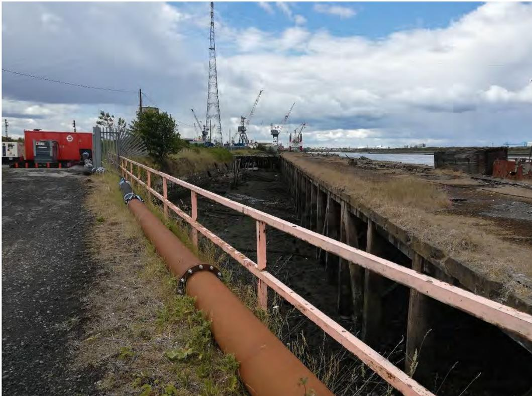
**Plate 9.2** The existing South Bank Wharf to be demolished, with the pumping station on the left. Minimal colonisation of the pillars supporting the deck of the wharf is evident.
